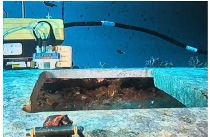
ACFM inspection of a pinhole support location
