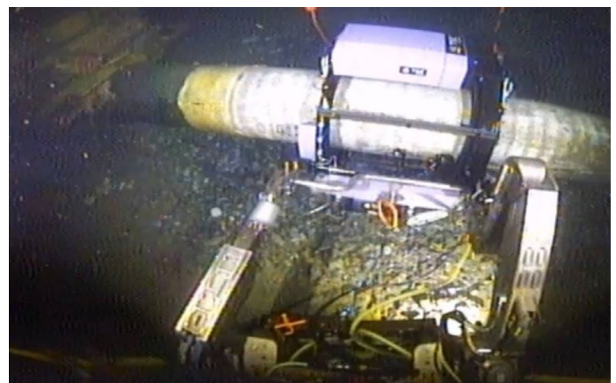
Pipeline with 0.3 mm FBE and 7.7 mm PP coatings
