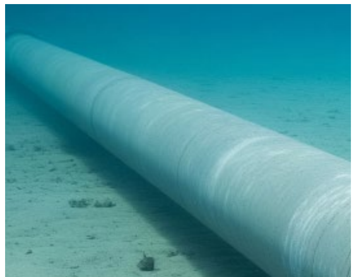
Subsea Pipeline with Concrete Weight Coat (CWC)
