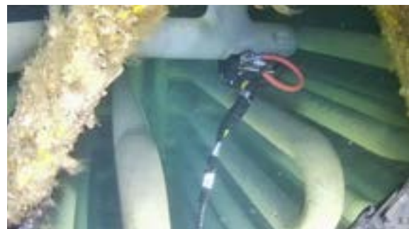
Wall thickness measurements
